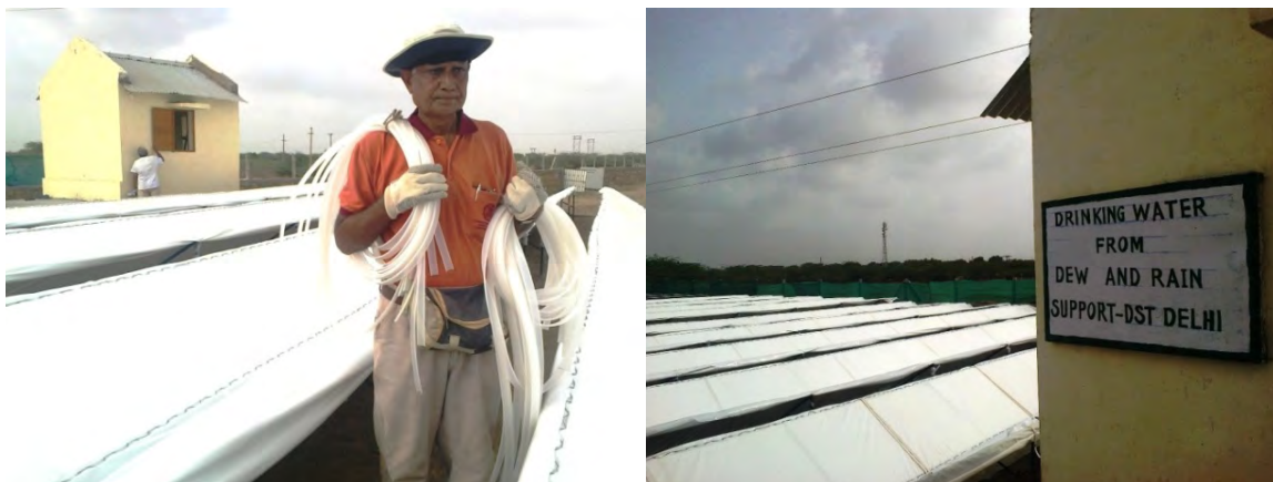
Dew Plant at Kothara village, Bhuj
